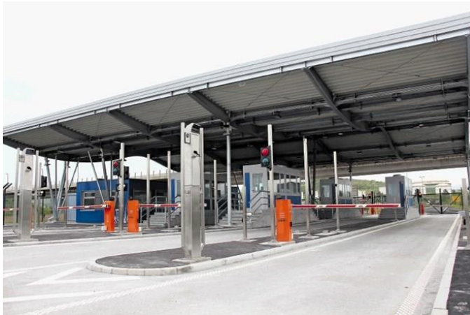
The new truck entrance to the port
