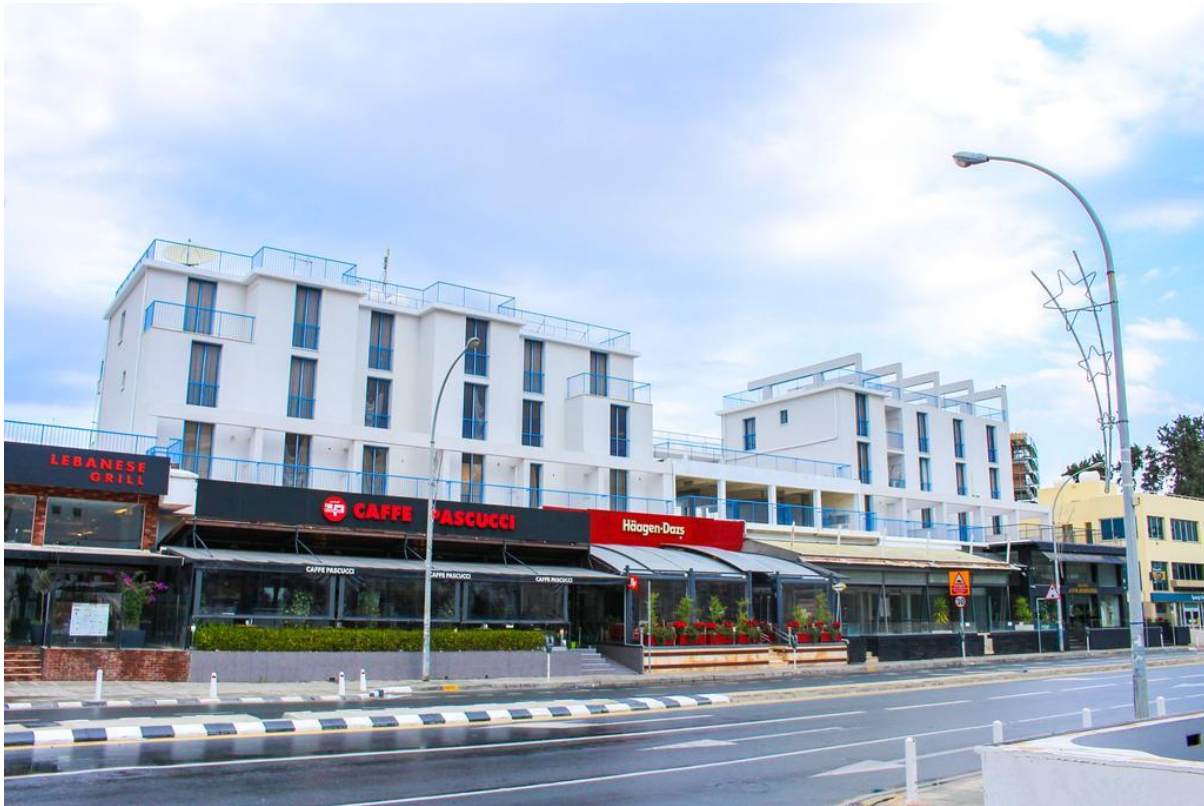
Busy road in Limassol (stretch without segregated cycle path in Germasogeia)
